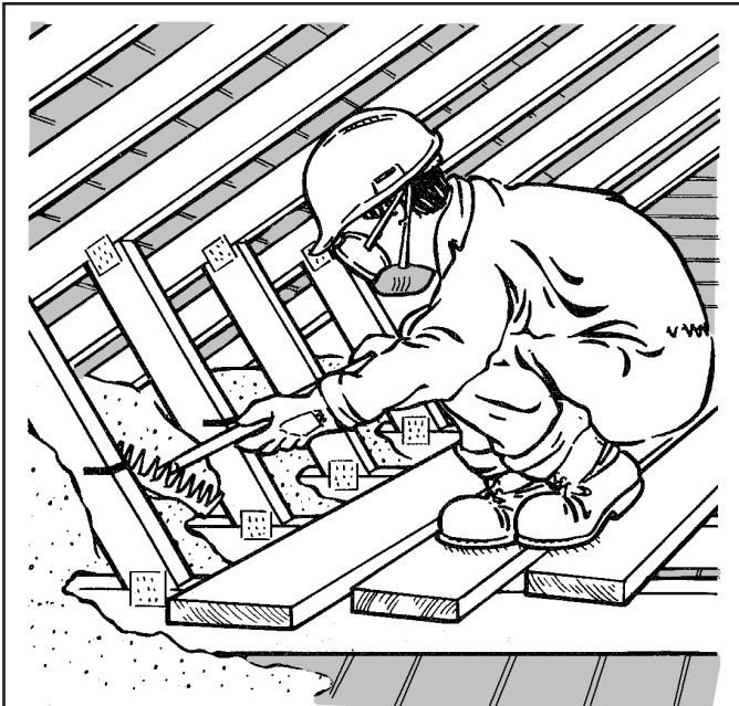
Installing loose-fill insulation (note the markers indicating final depth of insulation.)
